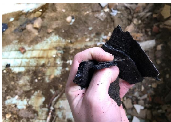
Obr. 3.86 Stav hydroizolace
