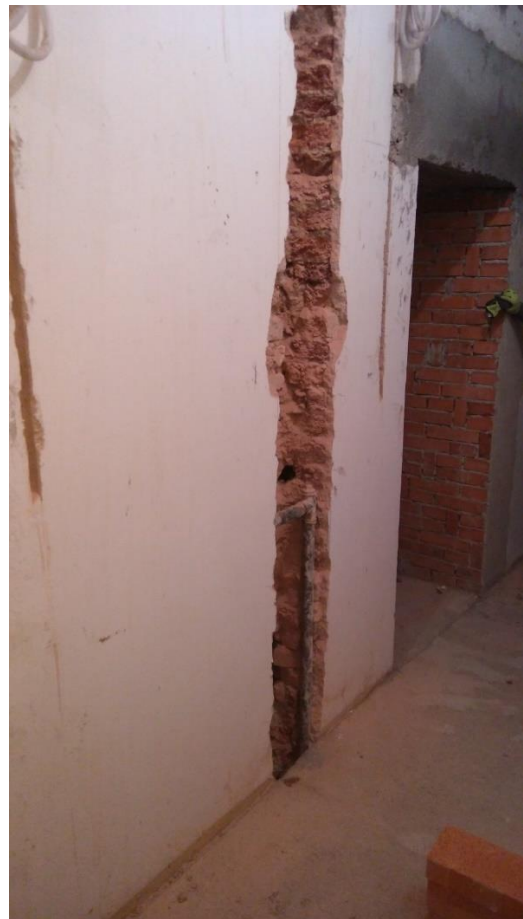
(Pic. 4: Installing the new Doorway next to the Chimney.)
