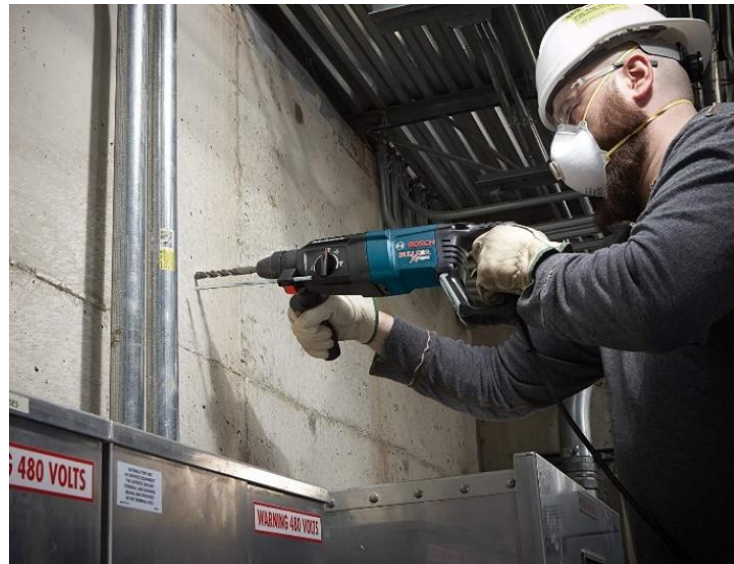
(Pic. 16. Drilling holes with long rod.)
