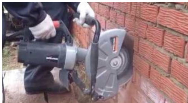
(Photo. 30. Cut the doorway opening.)
