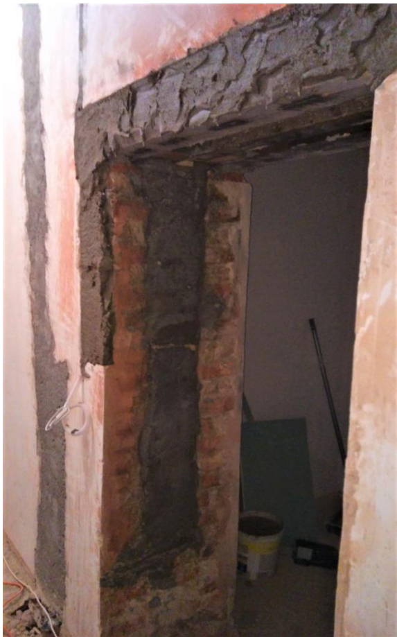
(Pic. 4: Installing the new Doorway next to the Chimney.)
