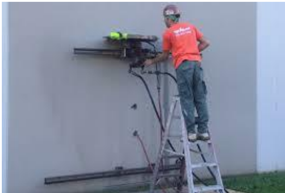
(Photo. 27. Cutting the wall with Mobile Circular Saw.)
