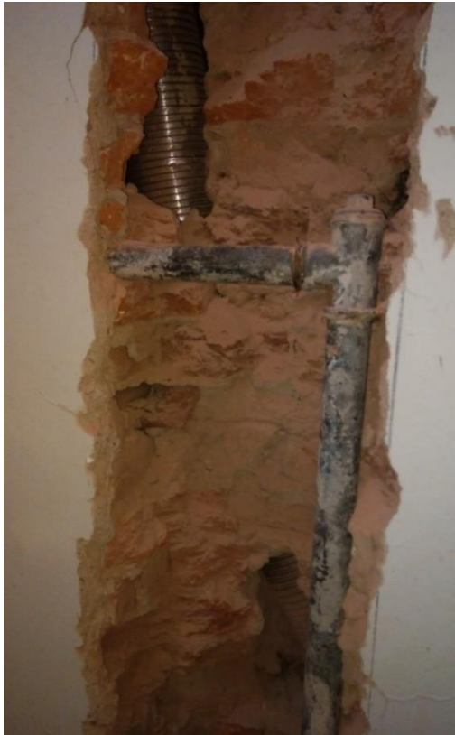
(Photo. 13.1 (on the left) and 13.2 (on the right). Stainless Steel Flexible Chimney Tube.)
