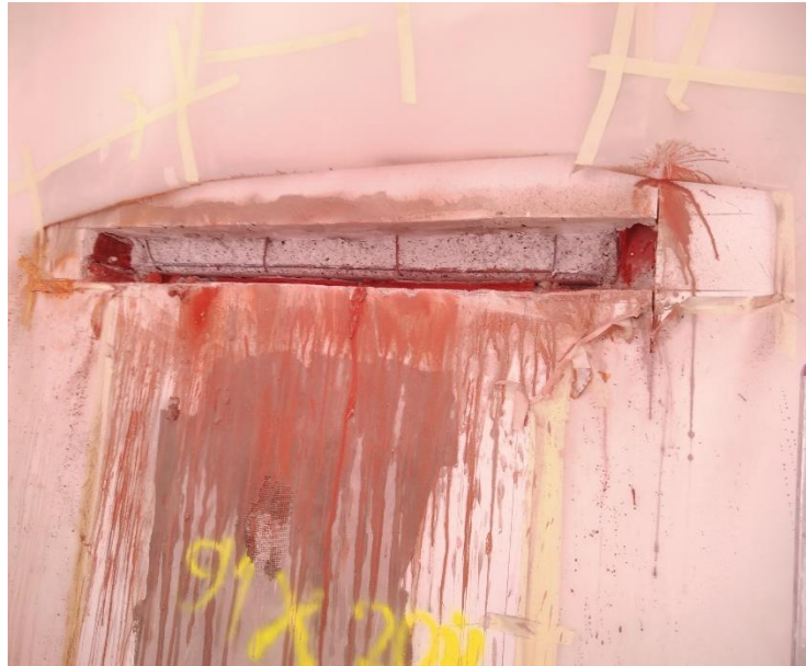
(Photo. 26. Prepared location for cutting a wall with Circular saw.)
