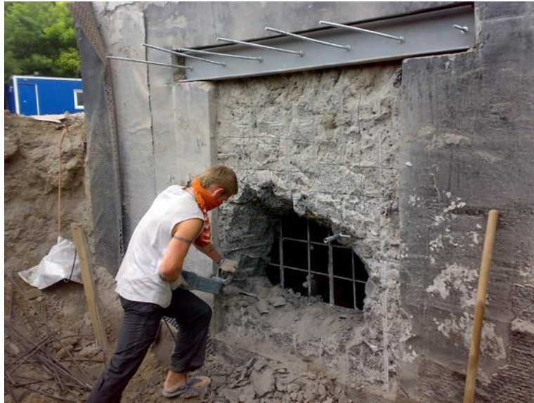
(Photo. 31. Demolition of the Doorway with perforator.)
