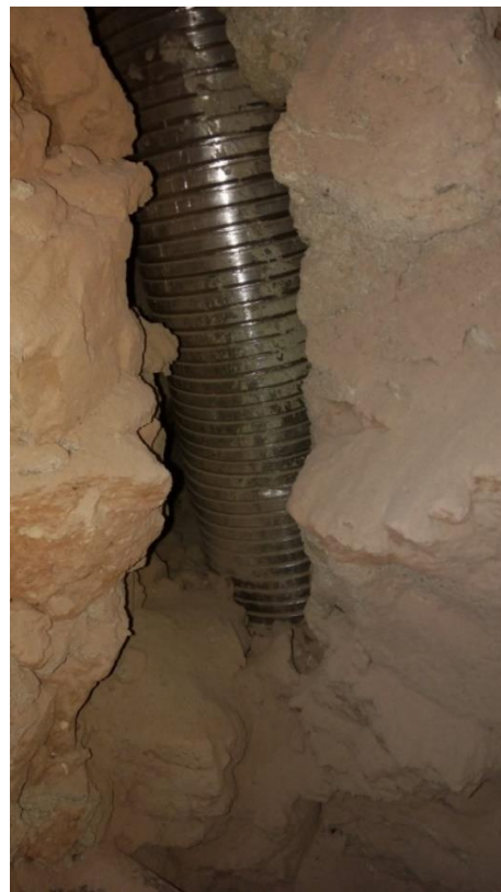
(Photo. 13.1 (on the left) and 13.2 (on the right). Stainless Steel Flexible Chimney Tube.)
