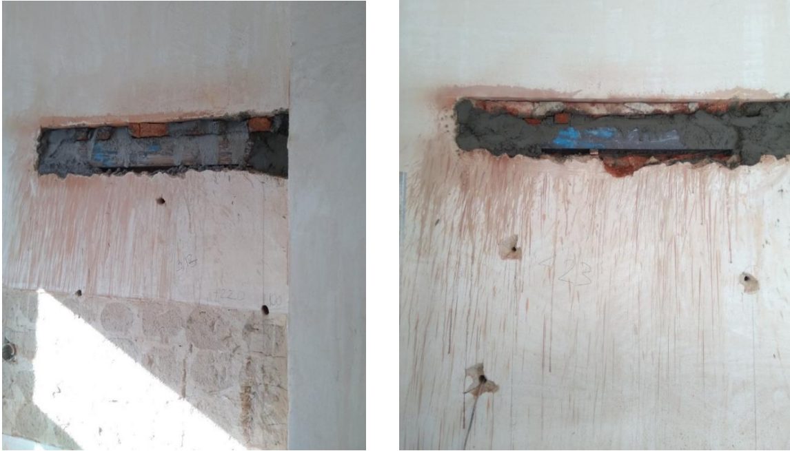
(Photo. 24. Drilling holes in the location of future doorway opening.)
