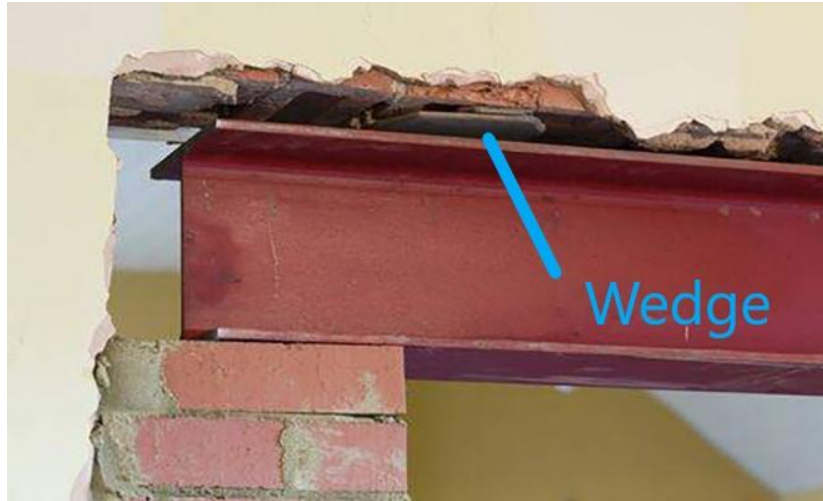
(Photo. 29. Underpinning of metal Lintels by wedges.)
