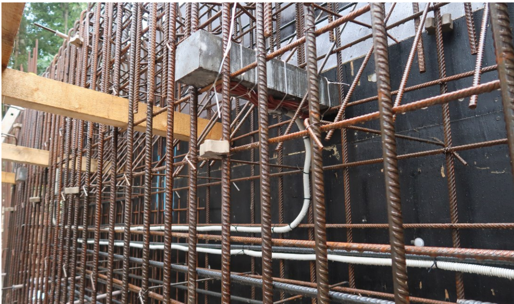
Figure 54 Installed casing beam with thermometers in abutment shaft. Branch box is placed on the bottom side of beam. Cables are led along reinforcement rods. (picture: P. Švecová)
