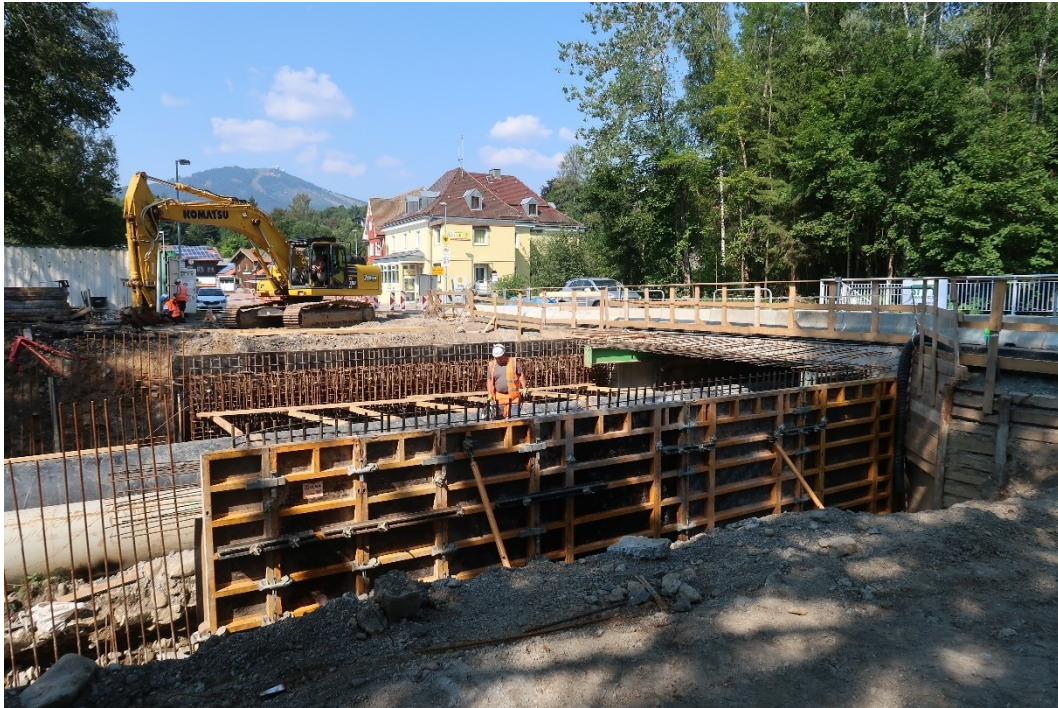
Figure 14 Bridge No. 27-117 under construction (picture: P. Švecová)
