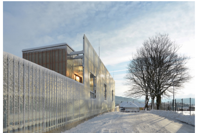
03 / street facade / winter
