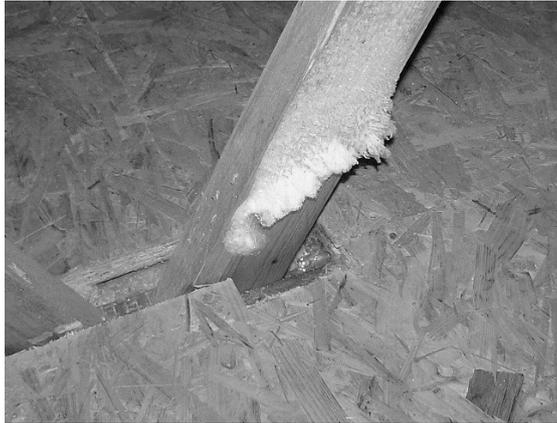
Fig. 2: frost accumulation on wooden truss above improperly sealed crack in the ceiling vapour barrier
