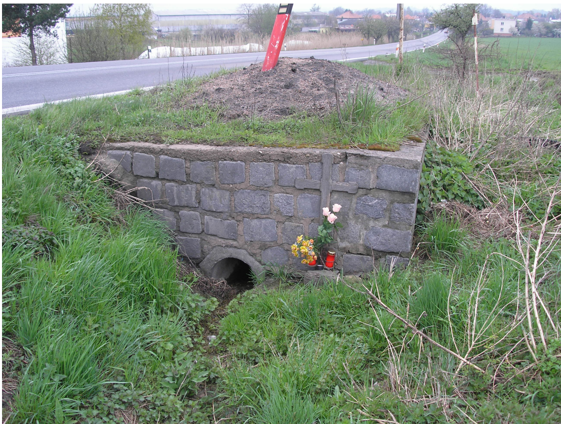
Figure 1.5: Example of a cross-drainage culvert. [1]
