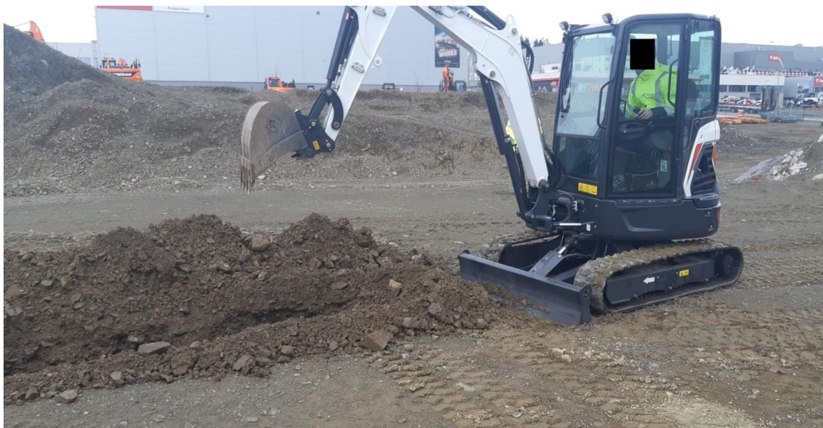
Figure 66 Excavator during the test
