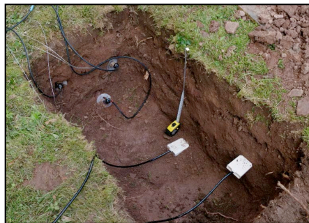
Figure 23 Detail of the shaft after installation of sensors
