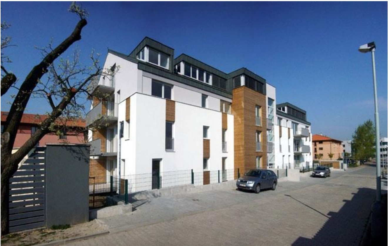
Figure 22: Existing residential building[26]
