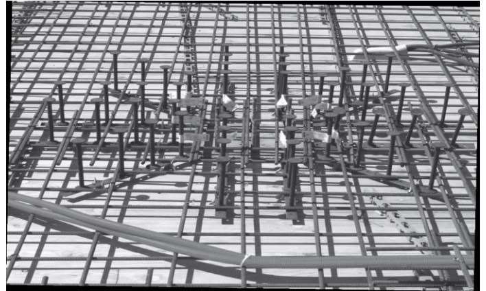
Figure 15: Shear reinforcement rail studs
