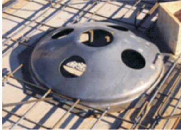
Figure 21: Flat slab with UFO punching preventer [22]
