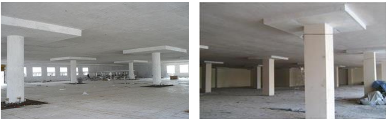
Figure 4: Reinforced concrete flat slab with drops
