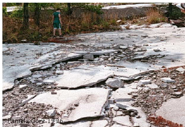
Figure 2.1: Pressure release causes the rock to break off into leaves or sheets along joints (from [4]).
