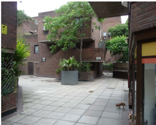
London: Greater London Council Architects Dep., Odhams Walk
