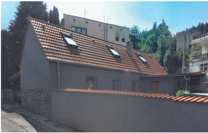
Fig. 1 Building 1 – the family house in Všenory (source: www.mapy.cz)
