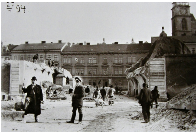
07 Demolition of Prague Gate /1894
