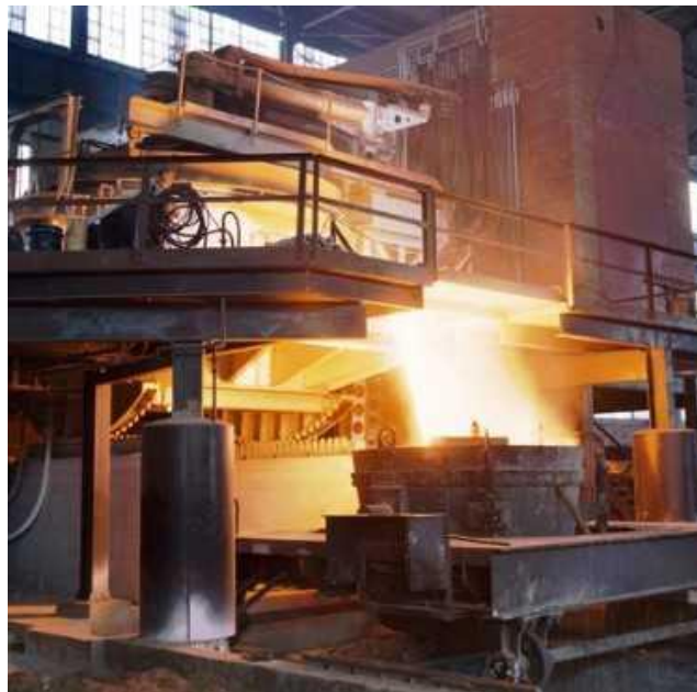
Figure 6: Electric arc furnace [17]
