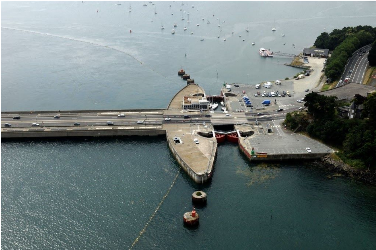
Figure 1.4.8 Rance Tidal Power Station
