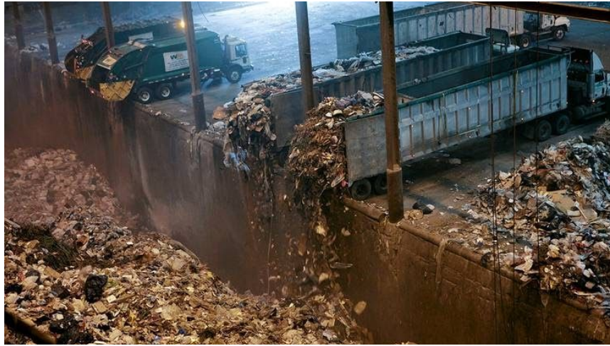
Figure 1.3.3 Trucks unloading waste to fuel storage groove in a MSW power plant, China.
