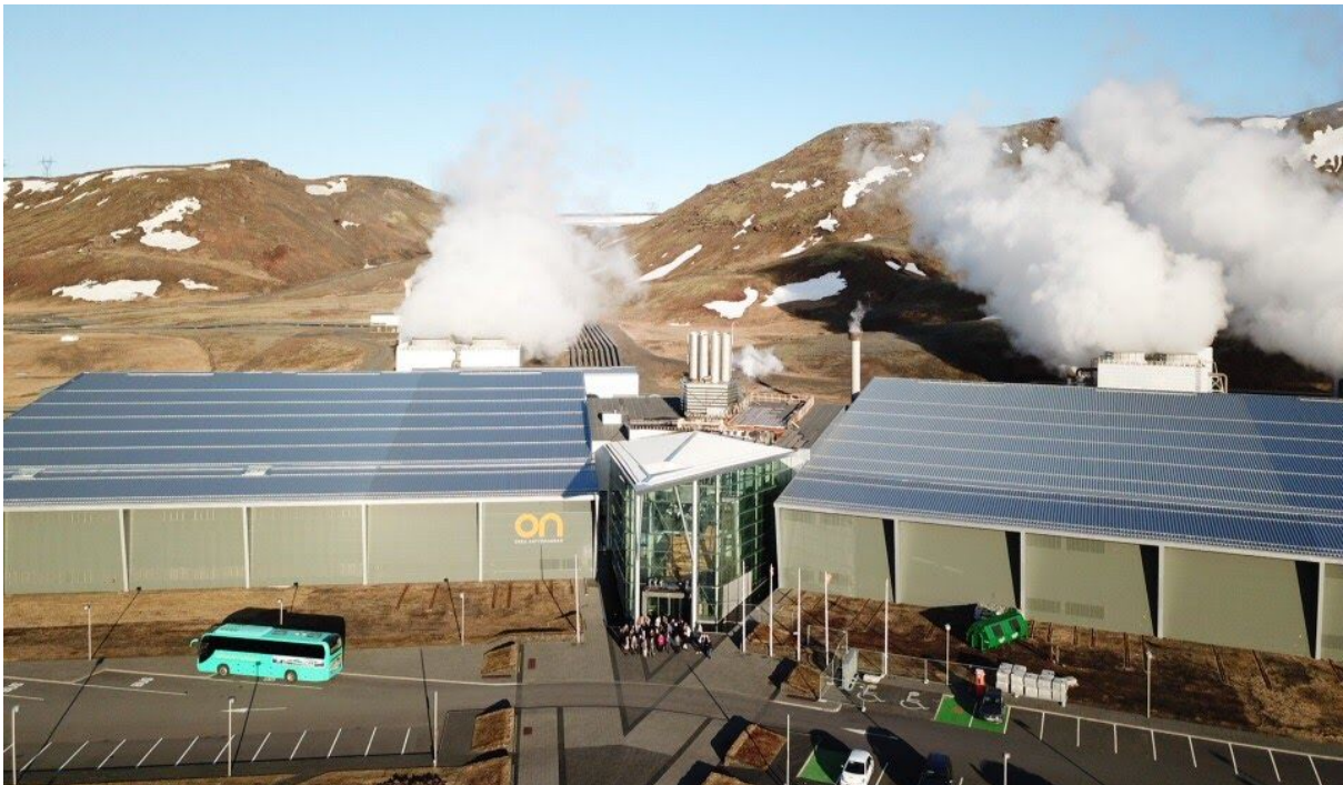
Figure 1.5.2 Hellisheidi Geothermal flash steam Power Plant, Iceland
