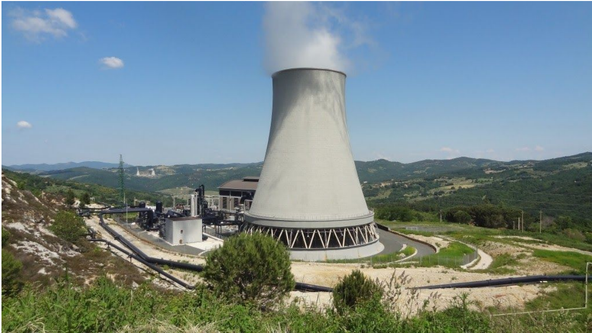
Figure 1.5.1 Larderello Geothermal Complex - dry steam geothermal power plant, Italy
