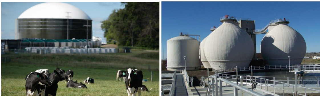
Figure 1.3.4 An anaerobic digesters at a dairy farm (left) and at the Nebraska wastewater-treatment facility, Lincoln, USA (right)
