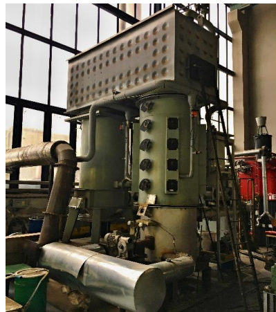
Figure 6: Photograph of the FBC boiler Golem
