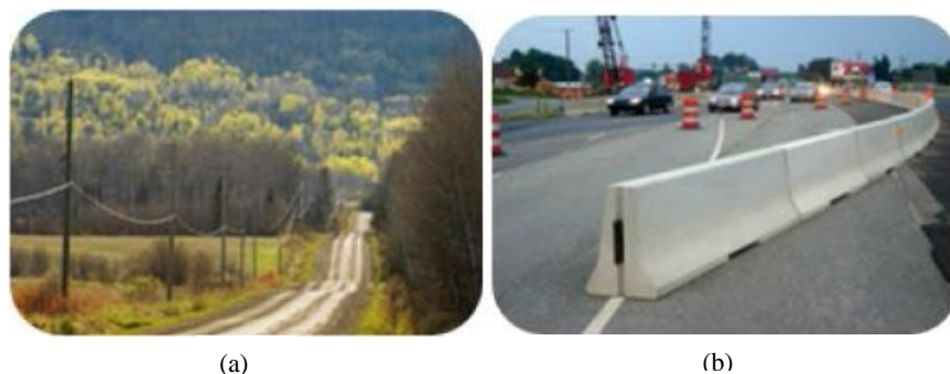
Figure 20: (a) Rural road; (b) Barrier and temporary cones 1
