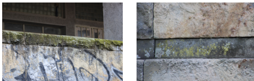
Figure 91 – Biofilm presence in North tribune.
