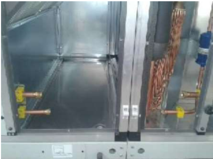
Connector is ready for connection to suction and discharge lines for with plate type recovery unit
