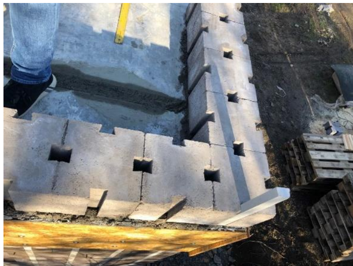
Figure 44 Setting of the corner block
