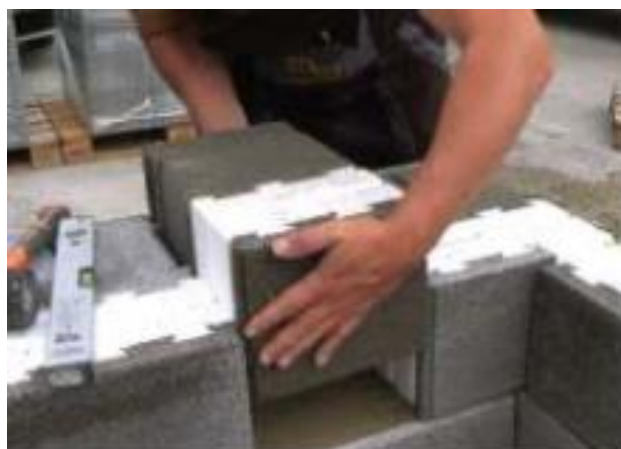
Figure 31 Livetherm block assemblying [30]
