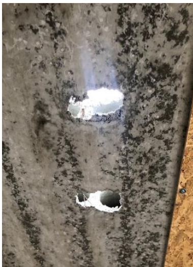
Figure 49 Hollow slab opening for communications
