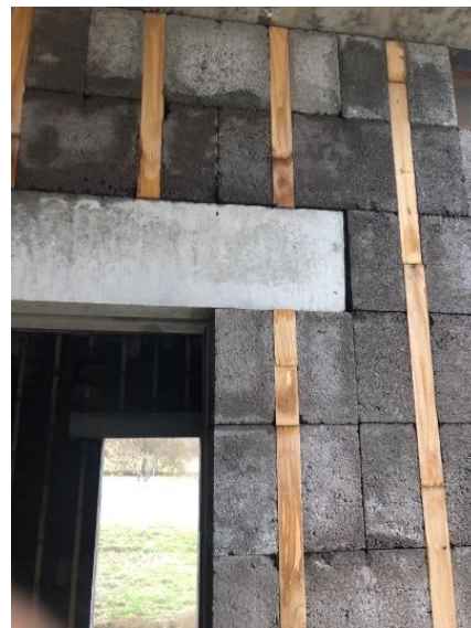
Figure 48 Wall construction with concrete lintel
