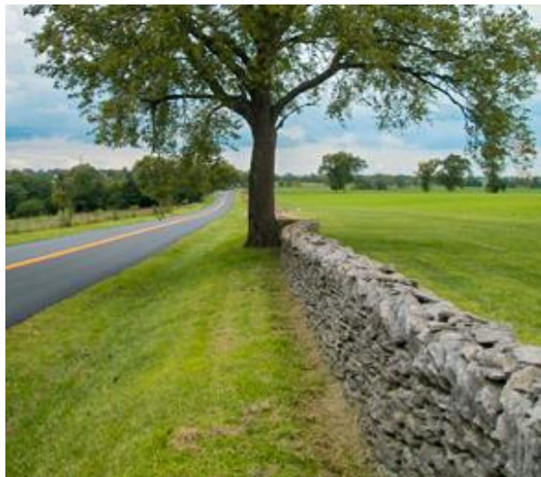
Figure 10 Rock fence made of limestone, central Kentucky[22]
