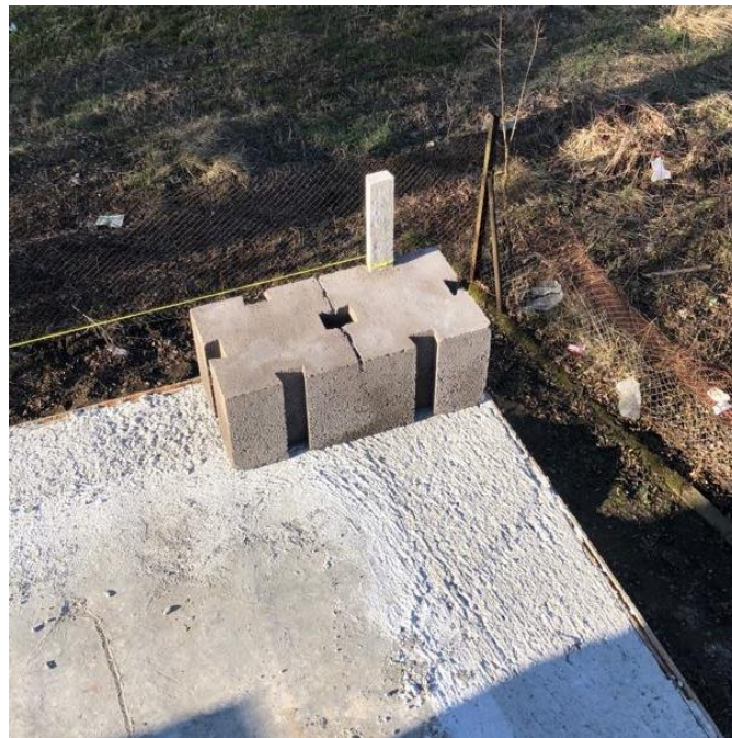
Figure 45 First course laid on mortar
