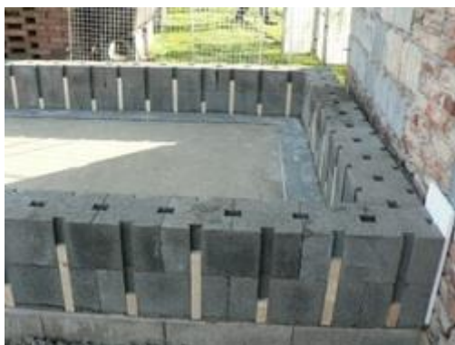
Figure 47 Position of the connection rails [2]
