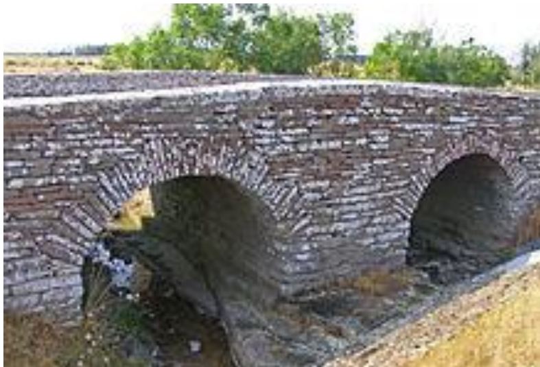
Figure 5 Medieval dry stone bridge in Alby, Sweden [17]
