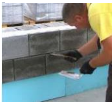
Figure 34 Manual pairing of blocks [30]
