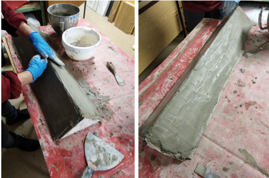
(Fig. 25: Concreting of interlayer. Source: Author)
