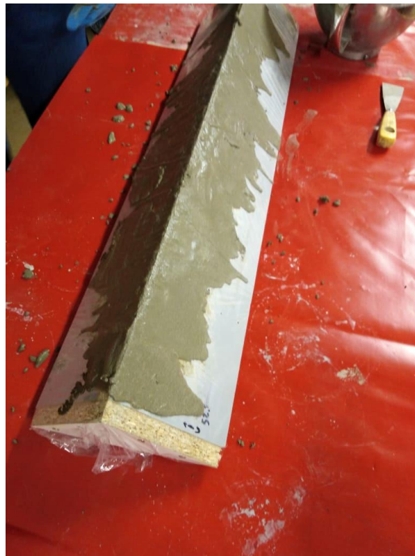
(Fig. 23: Concreting of the outer layer. Source: Author)
