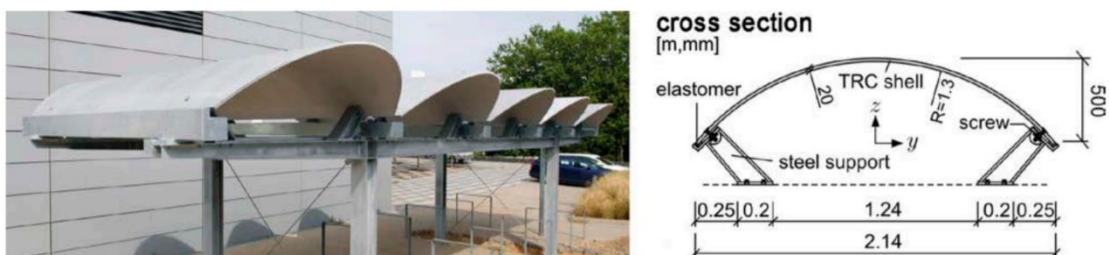
(Fig. 6: Roof of the bicycle stand made of laminated TRC barrel vault shells. Source: Edisciplinas.usp.br, 2019)
