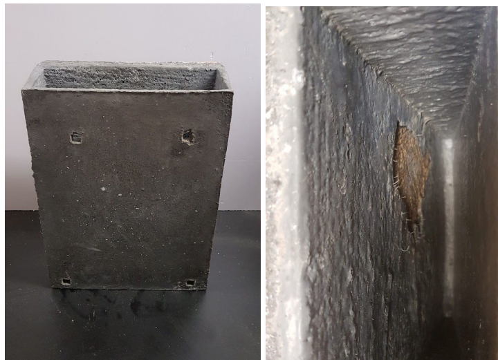
Fig. 27. Defects of Planter tile.
