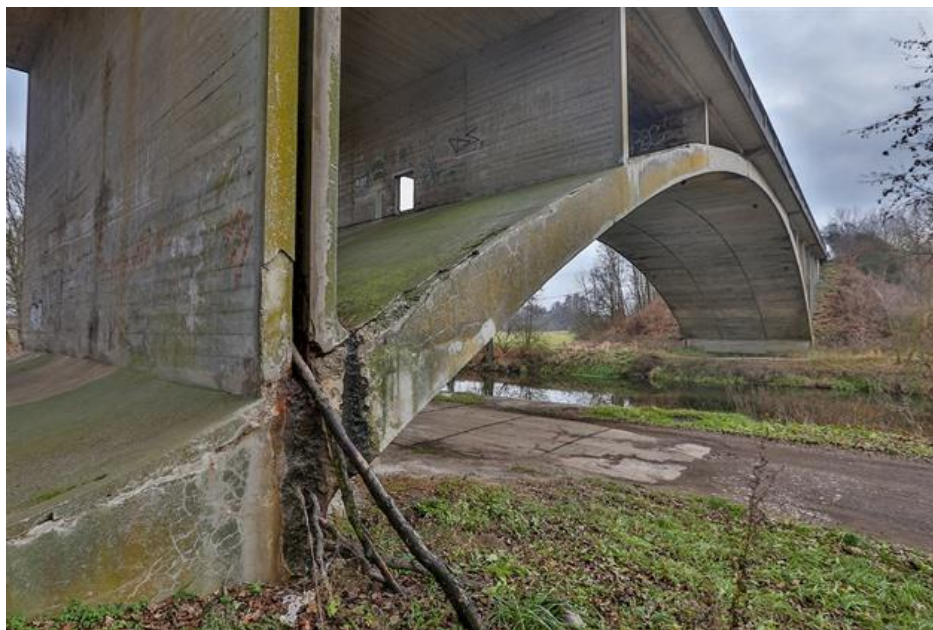
Obr. 12: Pohled na most [2.11]
