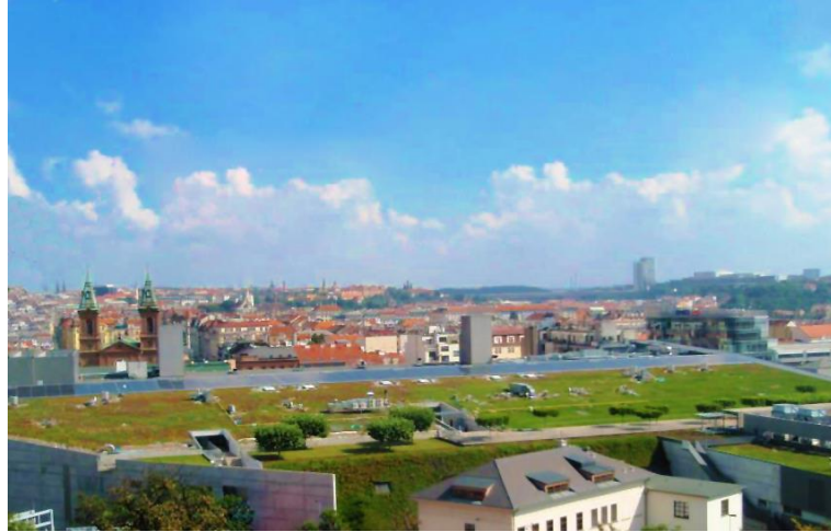
Figure 19: Extensive green roof of the shopping centre Novy Smichov, Prague
