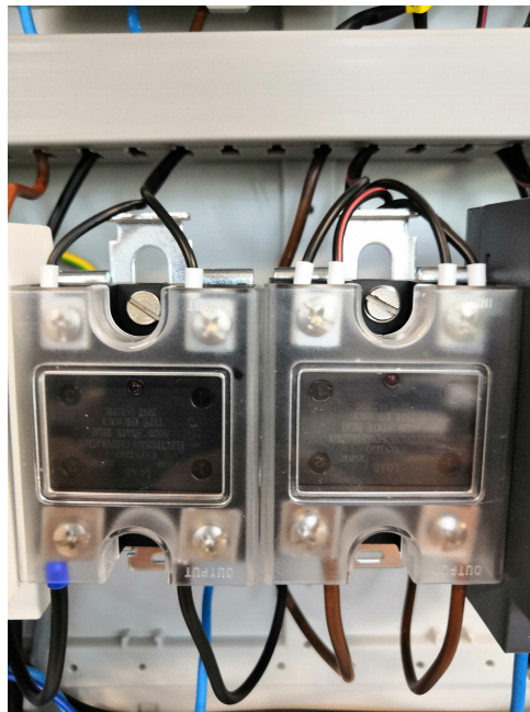
Figure 2.13: SSR relays for boiler
