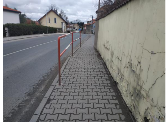
Figure 59 – Sidewalk narrowed down to a 1,0 m accompanied by railing (source: author)
