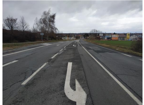
Figure 22 – Absence of traffic calming elements at the entrance to the municipality (source: author)
