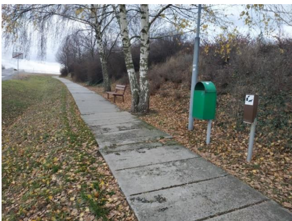
Figure 60 – Sidewalk lining the built-up area (source: author)
