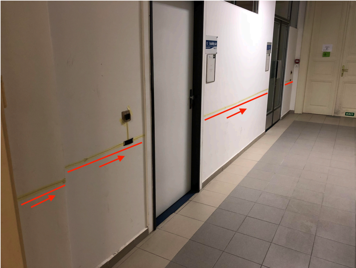
Figure 2.4: Concept of a guiding line, two mini-info buttons also visible above the line
