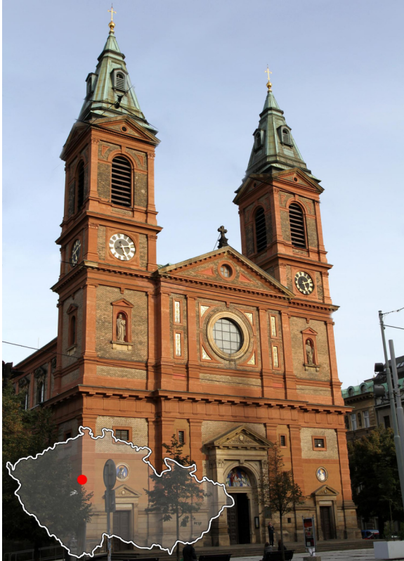
(a) Church front facade [50]
