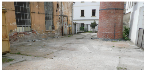
(a) Chimney location
