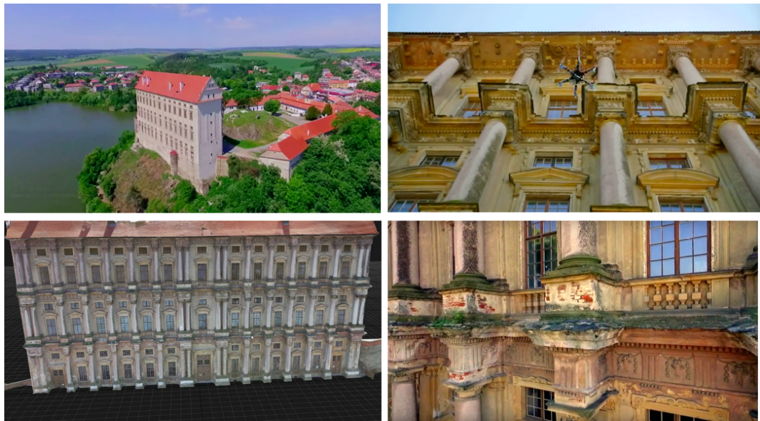
Figure 20: 3D modelling of a facade of Plumlov Castle within a project Dronument https://dronument.cz . Above: RGB pictures. Bottom: 3D models with a texture gained from captured images.
