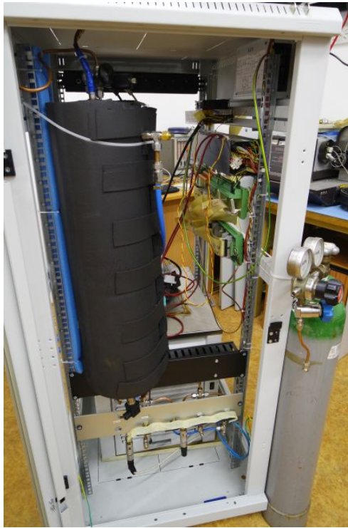
Figure 5.2: Constructed setup inside a rack
