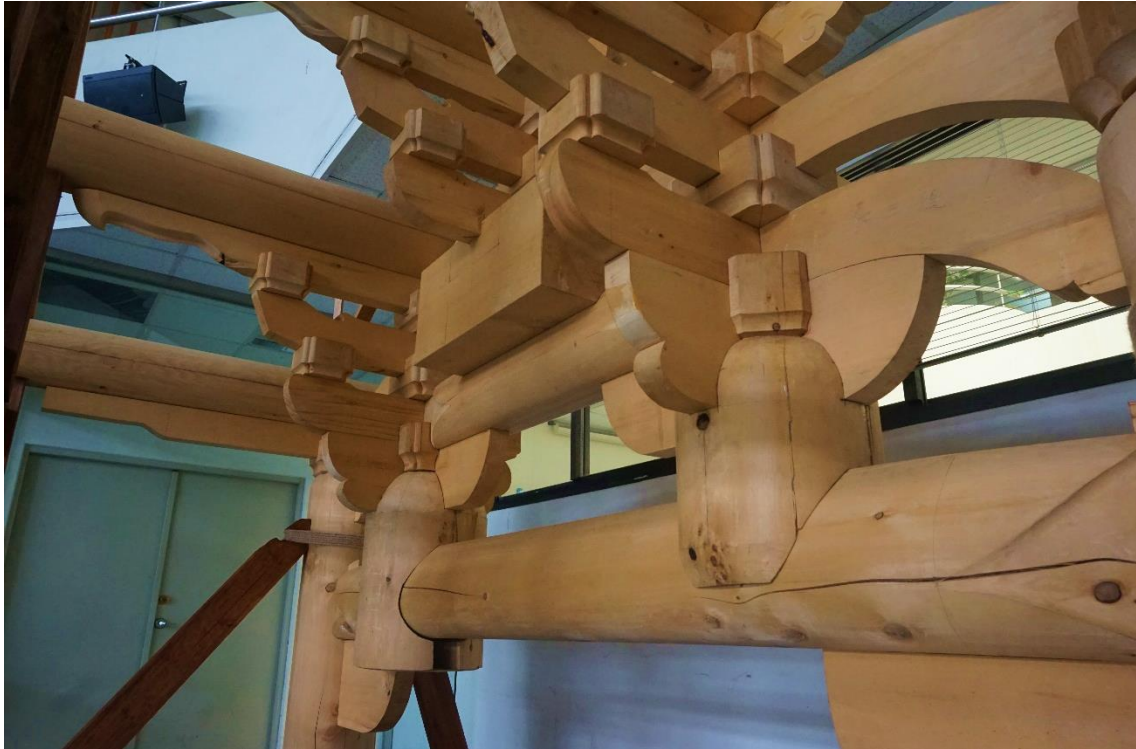
Pic. 15: Flexible wooden joint used in old Taiwanese temples, prevents from splitting and cracking built by Hsu Han-Chen (photo taken at the Department of Architecture at the NCKU in Tainan)
