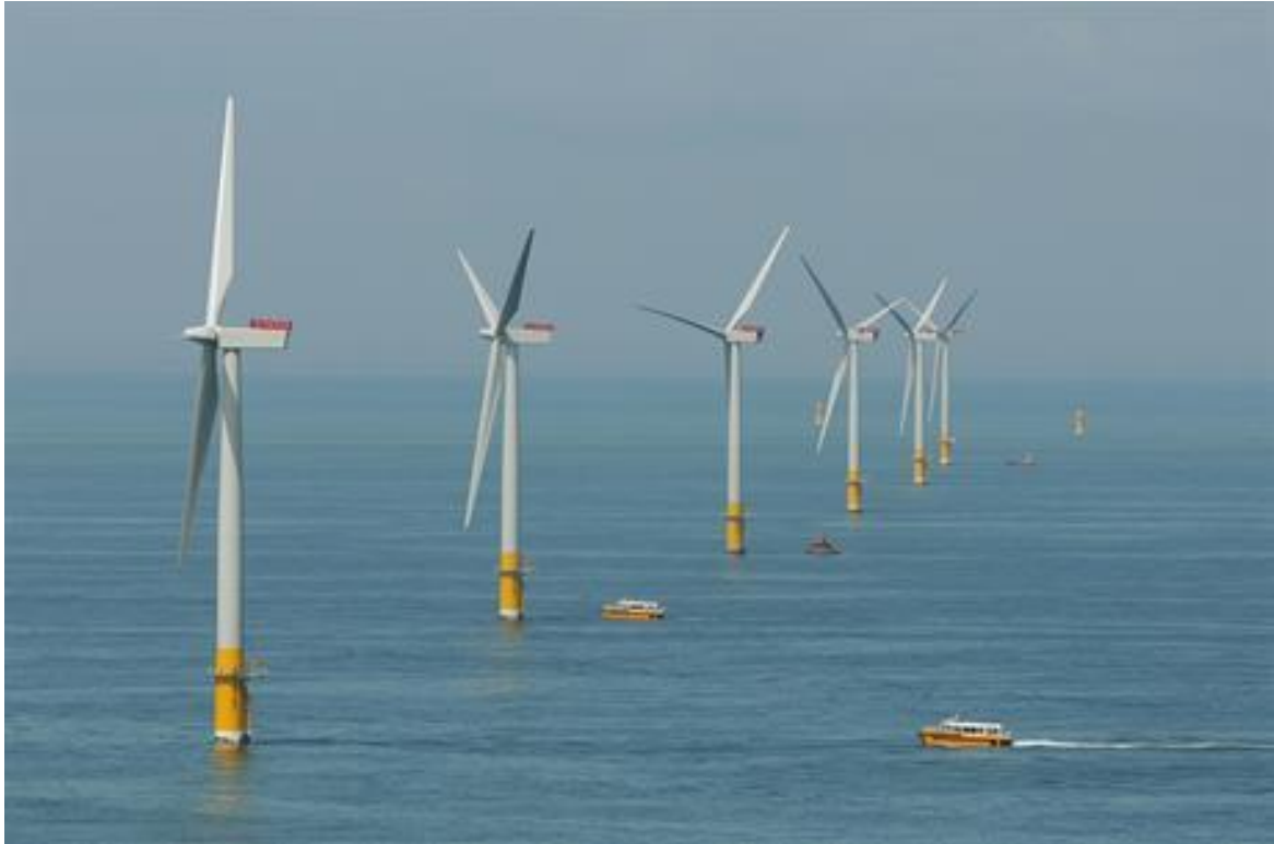
Figure 14 Greater Gabbard offshore wind farm
