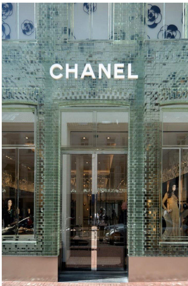
obr. 19: Průčelí Crystal Houses [27]
