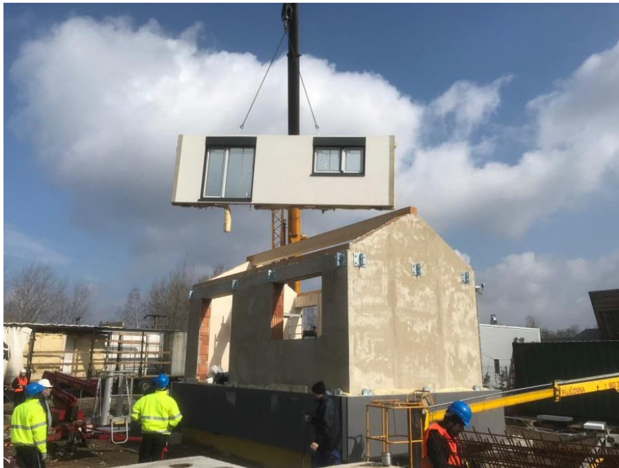
Figure 16: MORE-CONNECT demo building. Source: UCEEB
