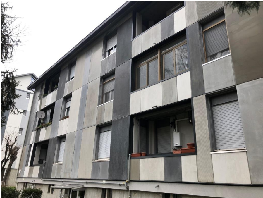
Figure 21: EASEE Italian demo building
