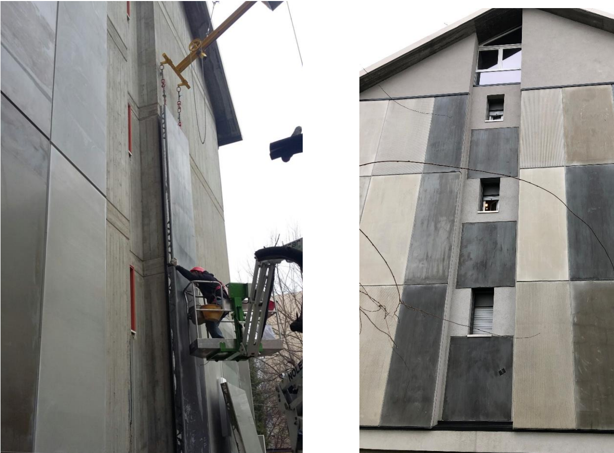
Figure 15, EASEE construction on the Italian demo building. Source: POLIMI elaboration
