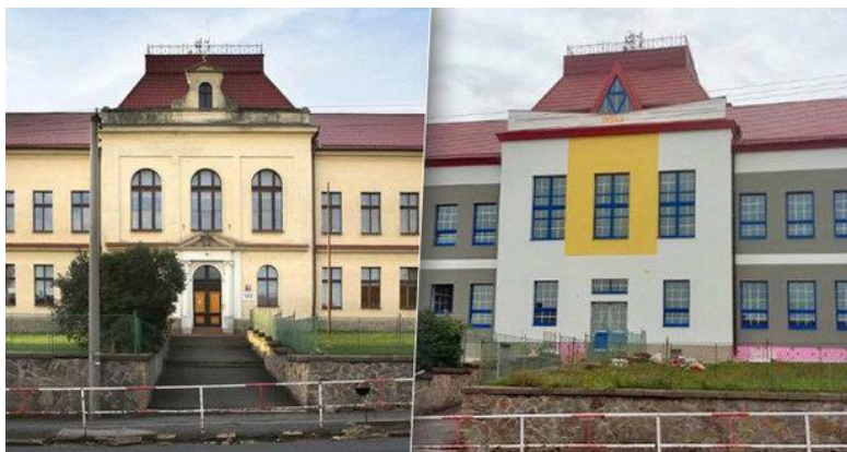
Figure 7: Unreasonably refurbished façade of a school, Source: iDnes.cz
