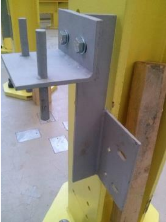
Figure 25: MORE-CONNECT facade anchor. Source:UCEEB
