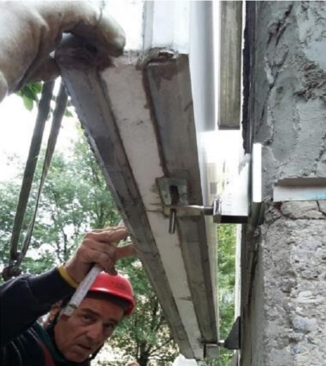
Figure 24: EASEE façade anchor. Source: POLIMI elaboration
