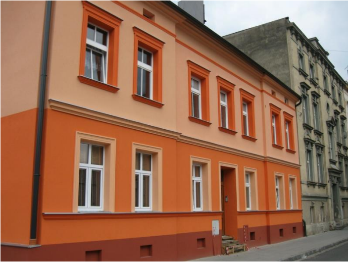
Figure 8: Detail façade refurbishment with ETICS. Source: Peter Hofer
