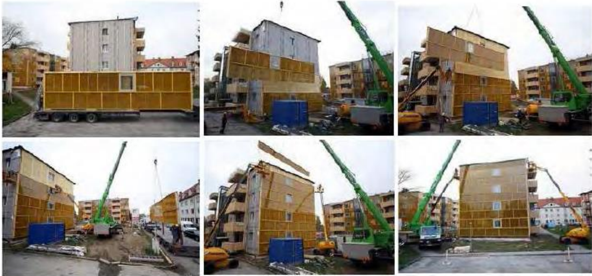
Figure 10: Assembling procedure of prefabricated façade modules within Dieselweg, Graz-Liebenau. Source: gap-solution
