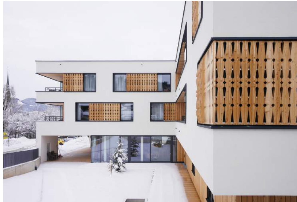
Retirement and Nursing Home Wilder Kaiser/SRAP Sedlak Rissland + Durschinger Architekten
