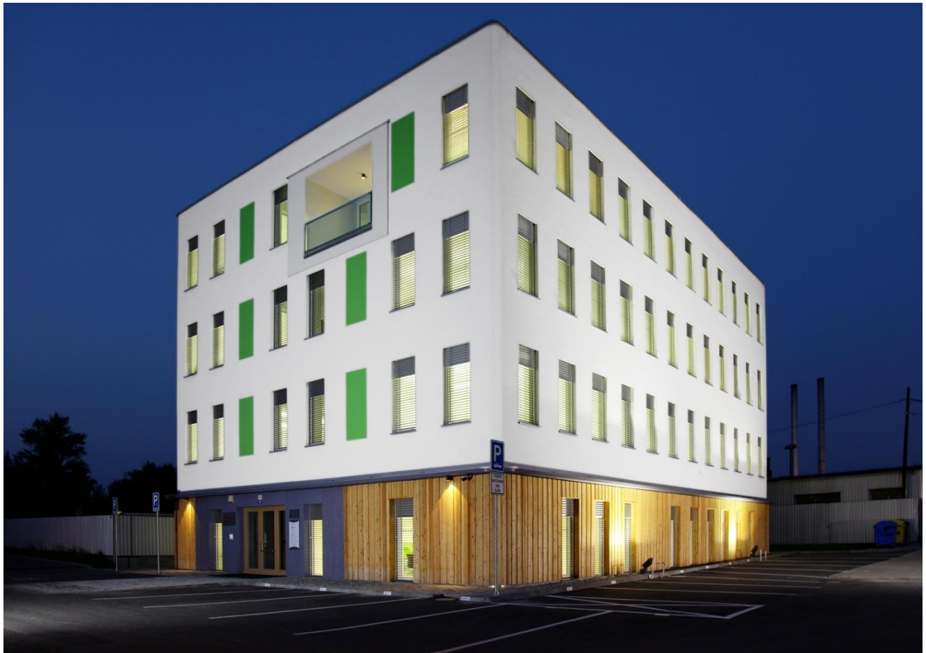
Figure 1. INTOZA passive office building
