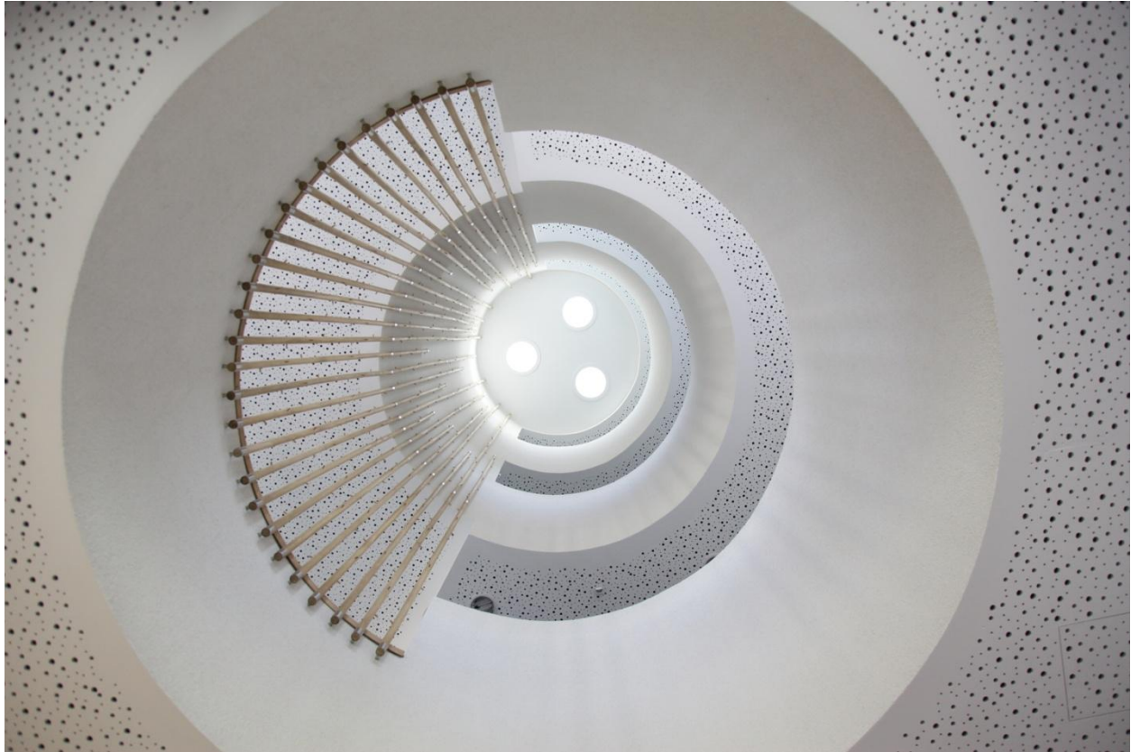
Figure 2. Opening in the slab
