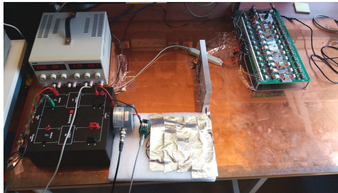
Fig. 75 The RPWI LVPS EMC test setup. Left top - bench power supply, left bottom - LISN, middle - wide bandwidth current probes, LVPS DUT and right - dummy loads board.
