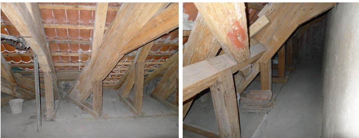
Figure 3.19 – The short columns connected to the rafters
