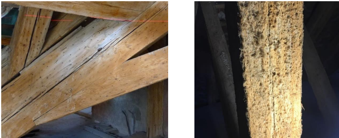
Figure 3.20 – The injection holes (left) and the fireproofing (right)
