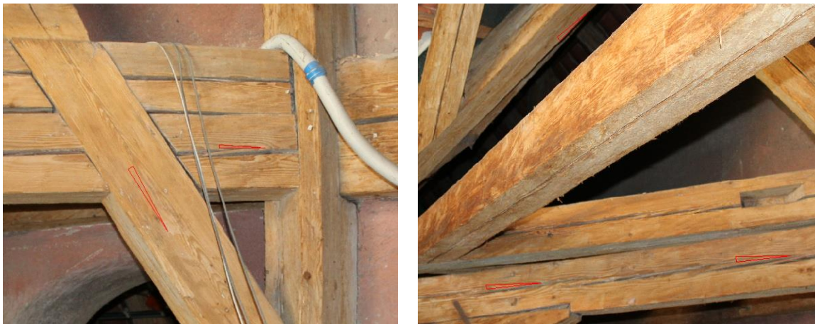
Figure 4.4 – The direction of the grains on Frame 1
