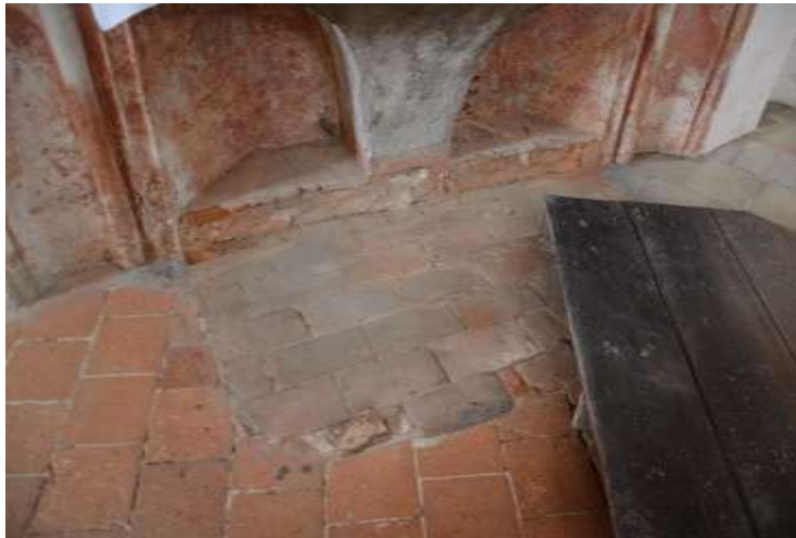
Figure 10- Replaced marble tiles of 36x36 cm dimension.
