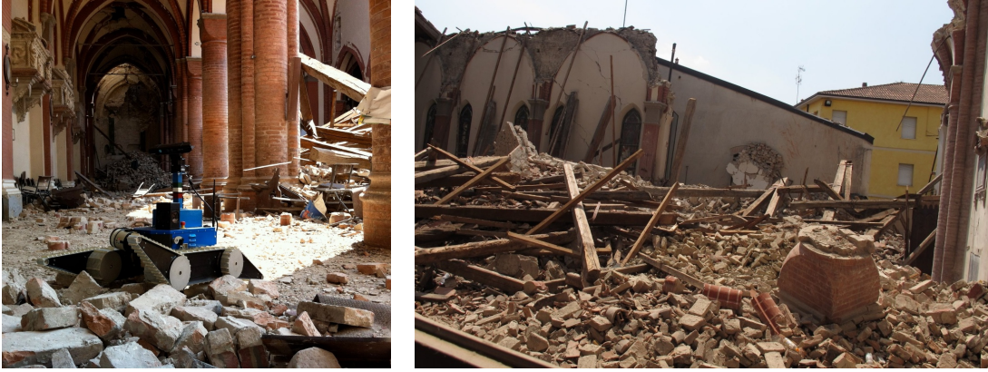
Figure 1.1. NIFTi ground robot exploring collapsed church in Mirandola, Italy, 2012. Wooden and stone debris, which filled its nave, are remains of its roof and ceiling.
