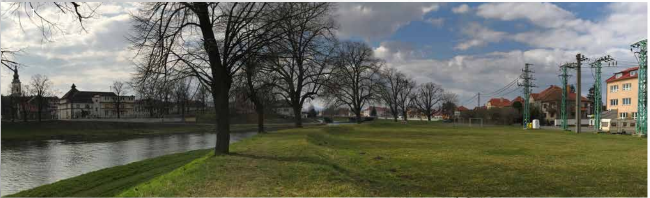
photo from the pedestrian path lined with full-grown linden trees towards the green area in front of the electricity distribution point
