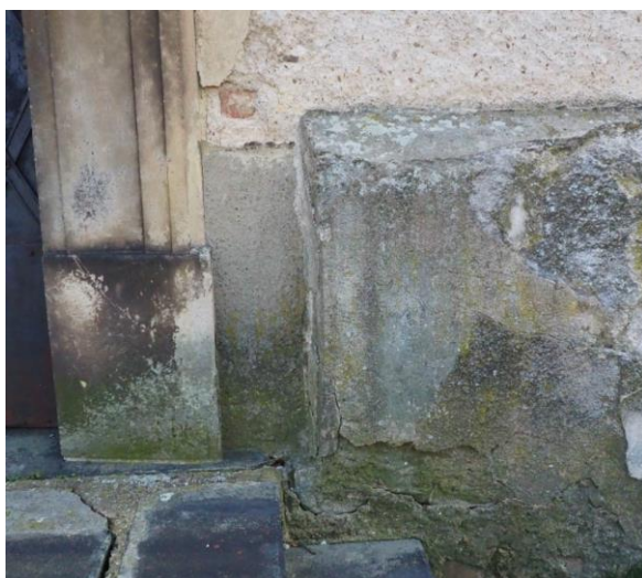
Obr.062 Biodegradace soklu
