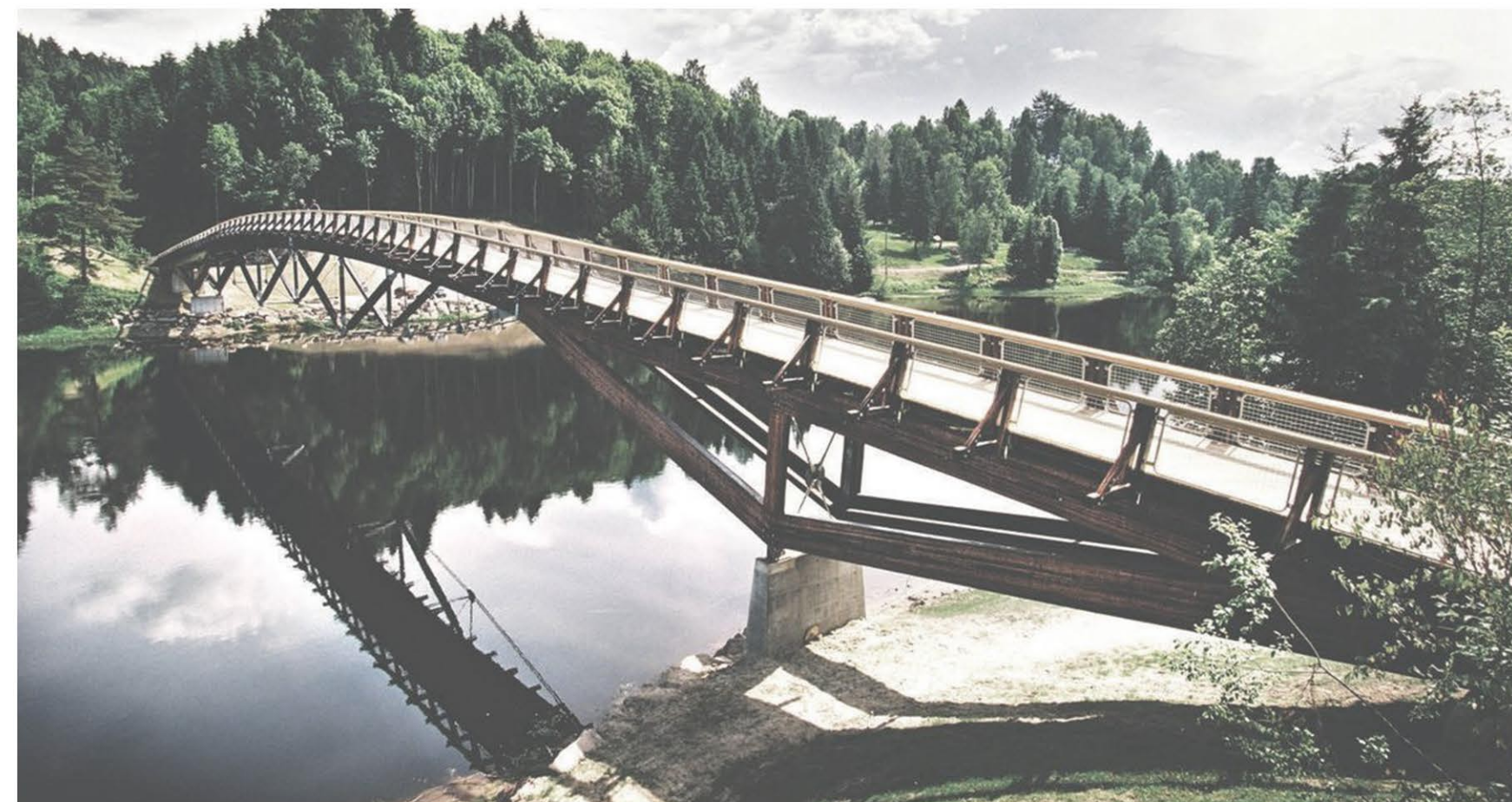
LARDAL BRIDGE, NORSKO
