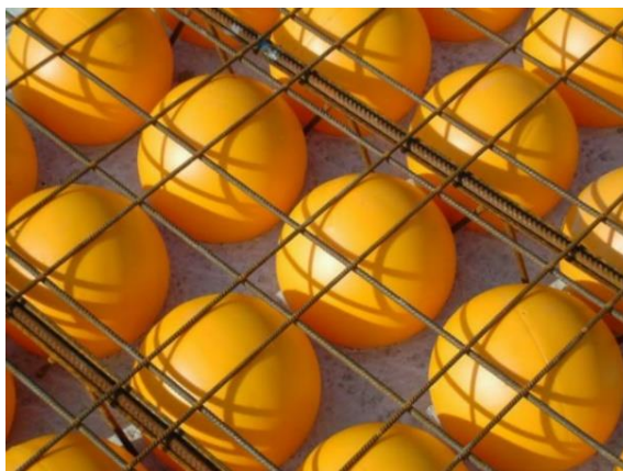
Obr. 2.8: Systém Bubble Deck [11]
