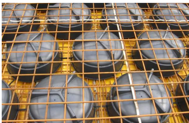
Obr. 2.18: Systém Beeplate [24]
