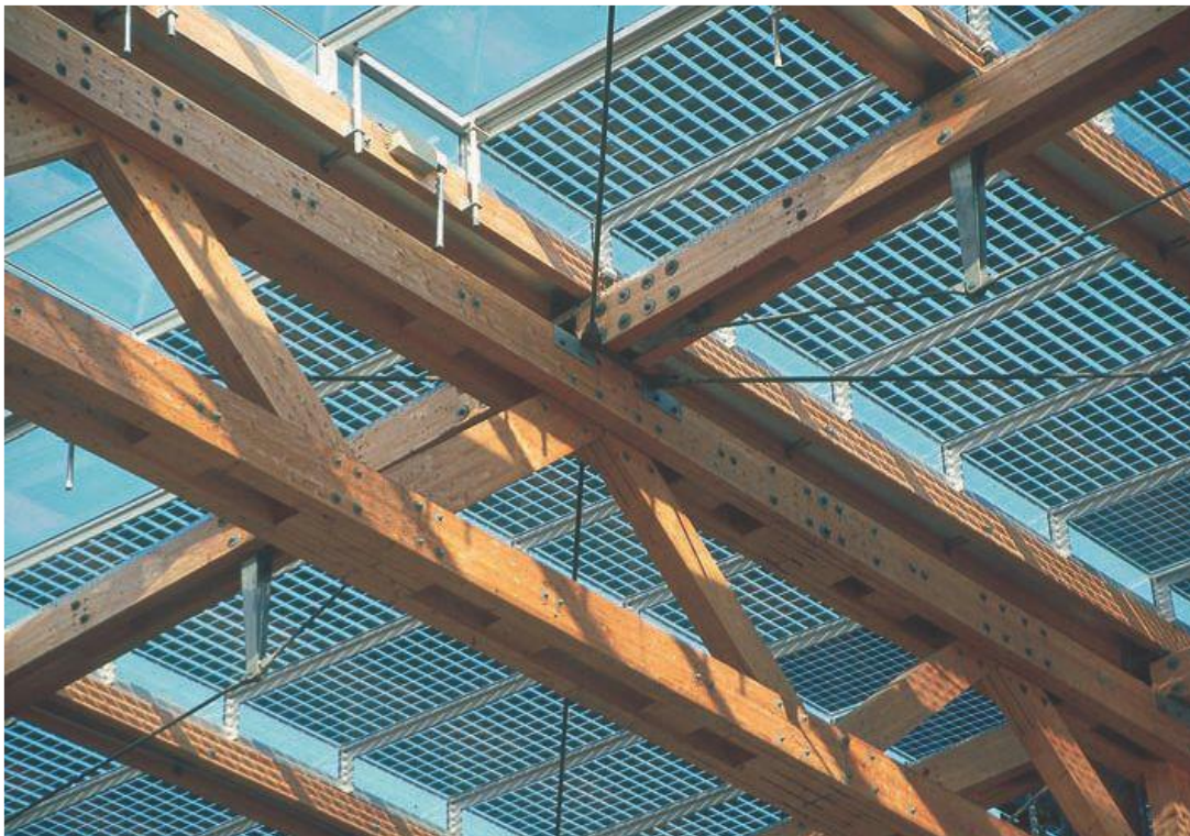
Figure 2.9: Photovoltaic cells located in the interlayer of laminated glass [1]
