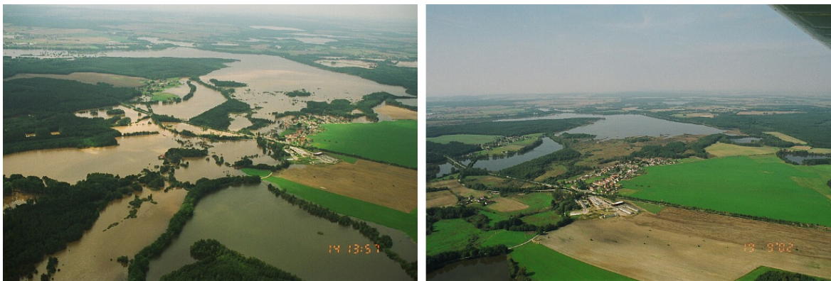
Figure 9.1: Retention of the Rožmberk pond during the flood in August 2002, MACR (2003)
