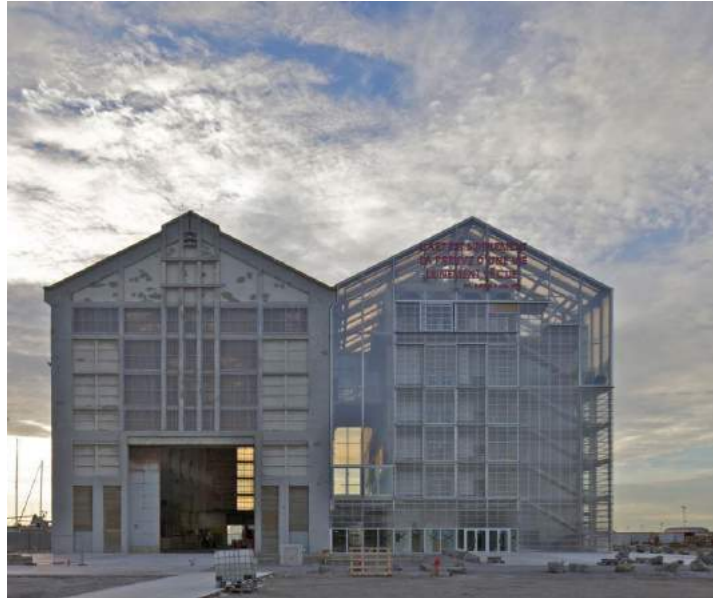
FRAC DUNKERQUE, Lacaton and Vassal, France
