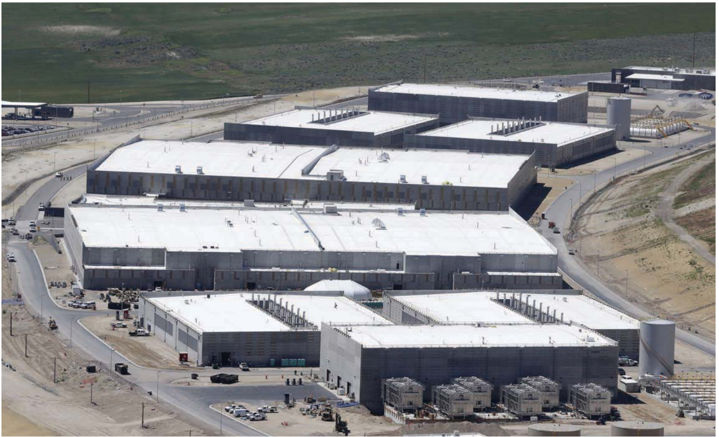
NSA Utah Data Center - June 2013 (fotografie AP/Rick Bowmer)
