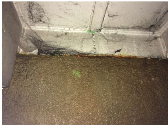
Picture 3-3 Left: signs of poorly compacted concrete, right: water leakage by expansion joints
