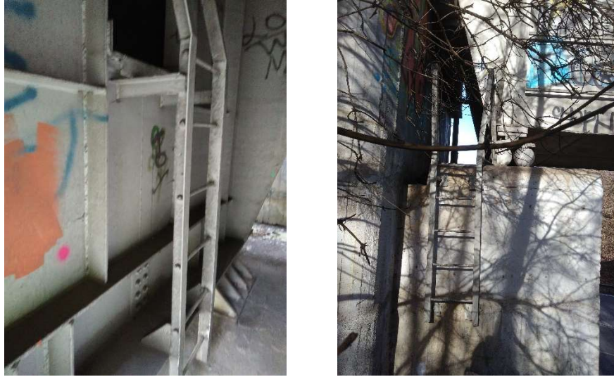
Picture 5-3 - maintenance ladders
