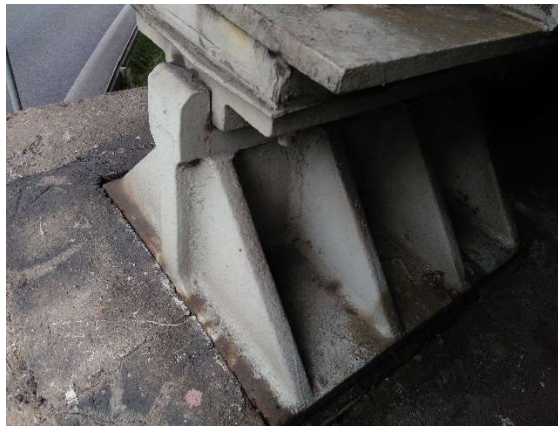
Picture 2-3 - fixed bearing (type II-P-5)
