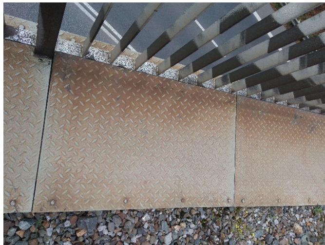
Picture 5-2 - detail of maintenance walkway
