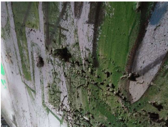
Picture 3-3 Left: signs of poorly compacted concrete, right: water leakage by expansion joints
