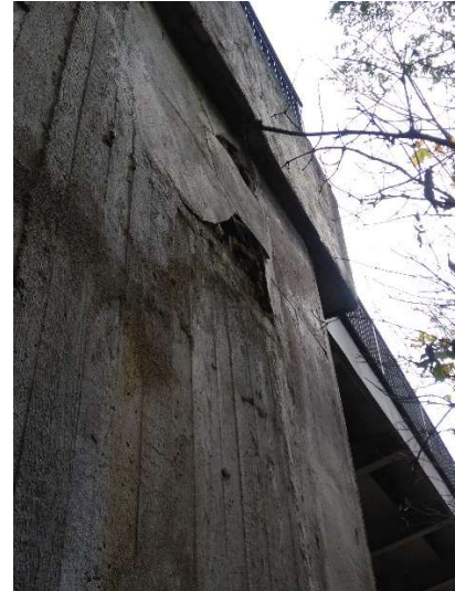
Picture 3-1 – bulging wing walls – abutment S1 on the left side and S2 on the right side
