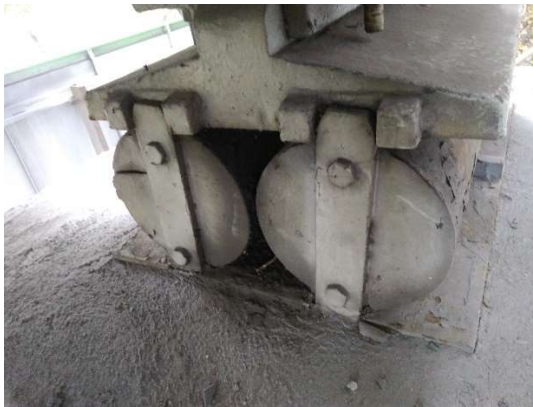
Picture 2-4 - expansion bearing (type II-V-5)
