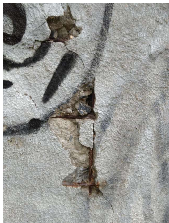
Picture 3-2 - water leakage and vertical crack on abutment S2
