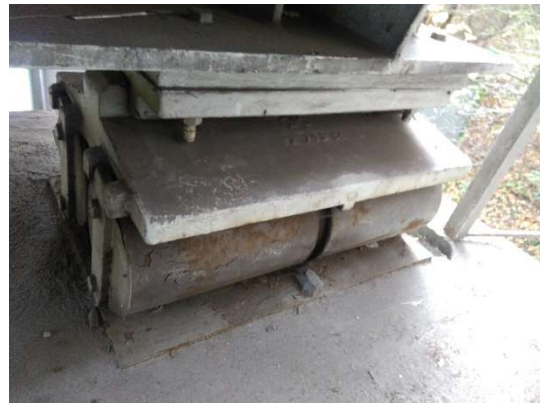
Picture 2-4 - expansion bearing (type II-V-5)
