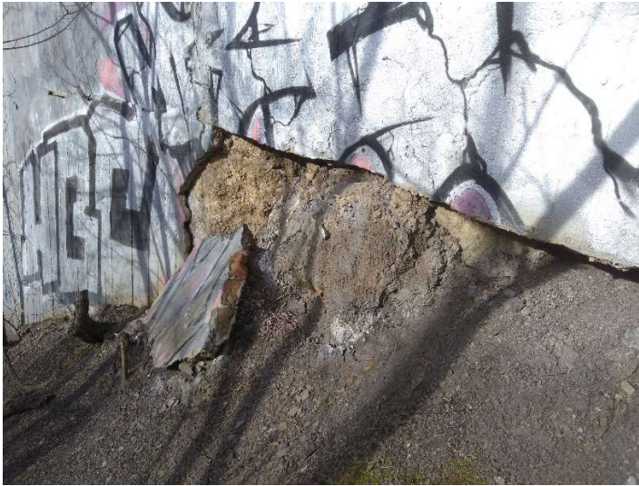
Picture 3-1 – bulging wing walls – abutment S1 on the left side and S2 on the right side
