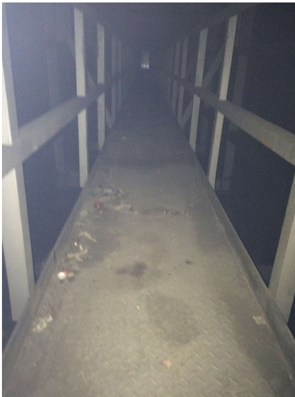
Picture 2-2 - inspection walkway inside a bridge
